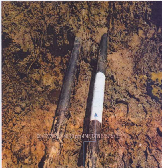
REPAIR POINT (WRAPPED)
