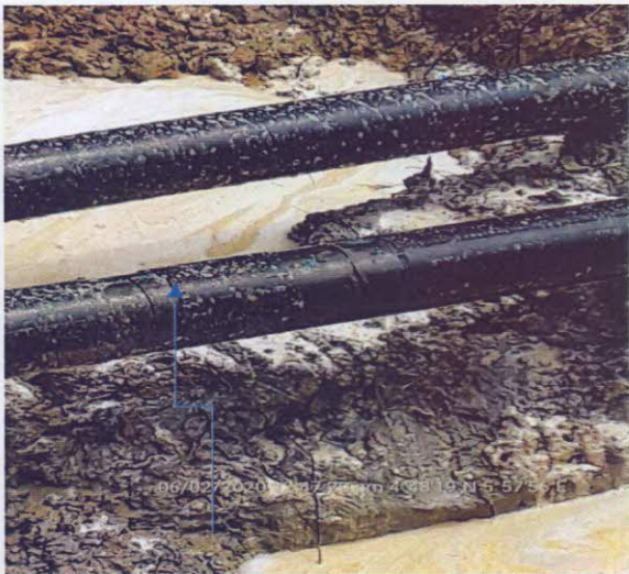
SPILL POINT (AFTER EXCAVATION) HACKSAW CUTS
